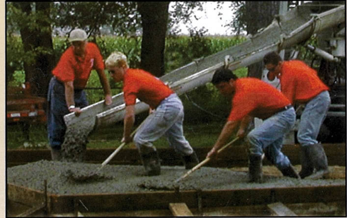
All our buildings start with a professionally finished Concrete Floor .
